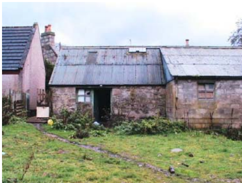
Fig. 2 : Partial exterior view of steading
