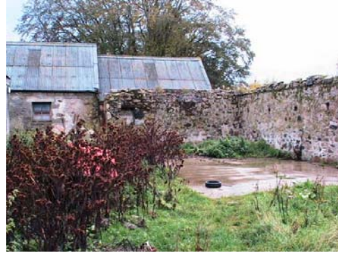
Fig. 13 : ruins of buildings and garden ground.
