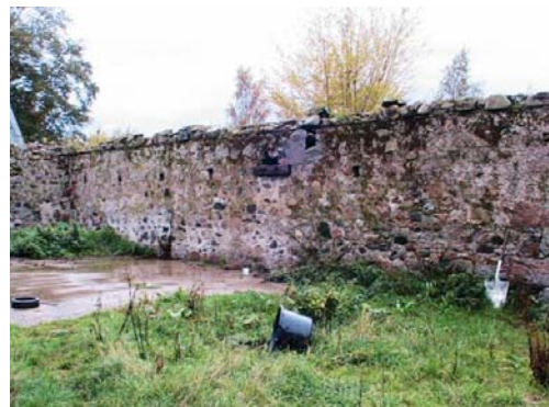
Fig. 5 : Ruins of former barn
